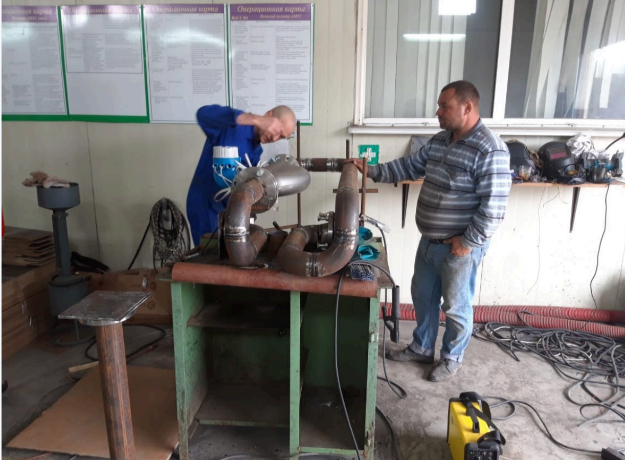
Welding pipes by templates in the workshop
